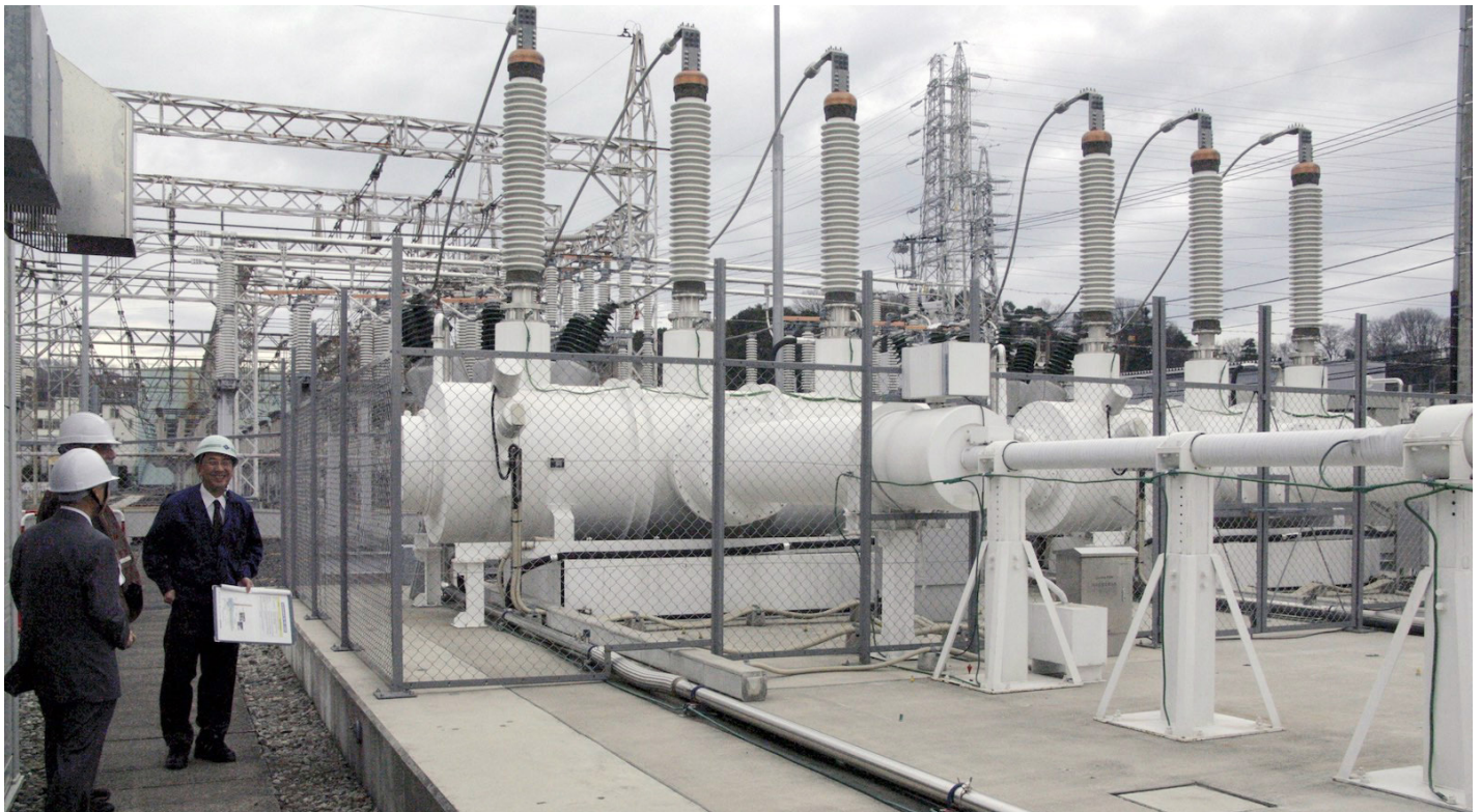
Superconducting cable terminations at the Asahi Substation in Japan. Image courtesy of Steve Eckroad.
