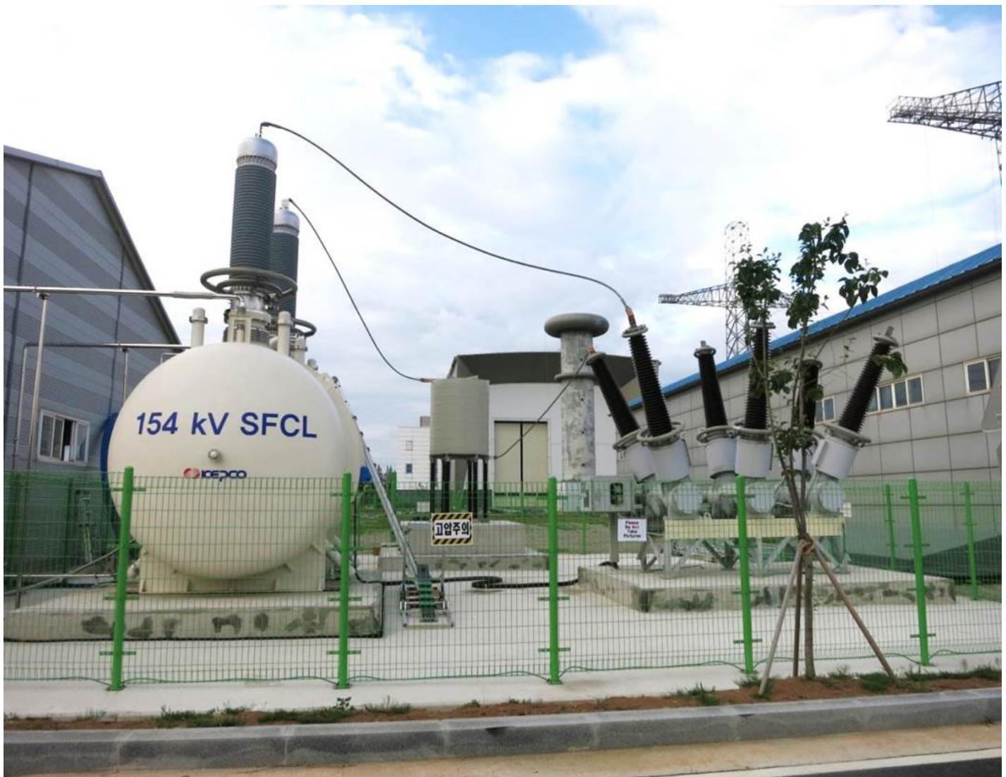
154 kV SFCL in Gochang Korea. Image courtesy of KEPCO.
