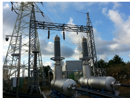
End of termination of 80kV DC HTS Cable in Jeju Island, Korea. Image Courtesy of KEPCO.
