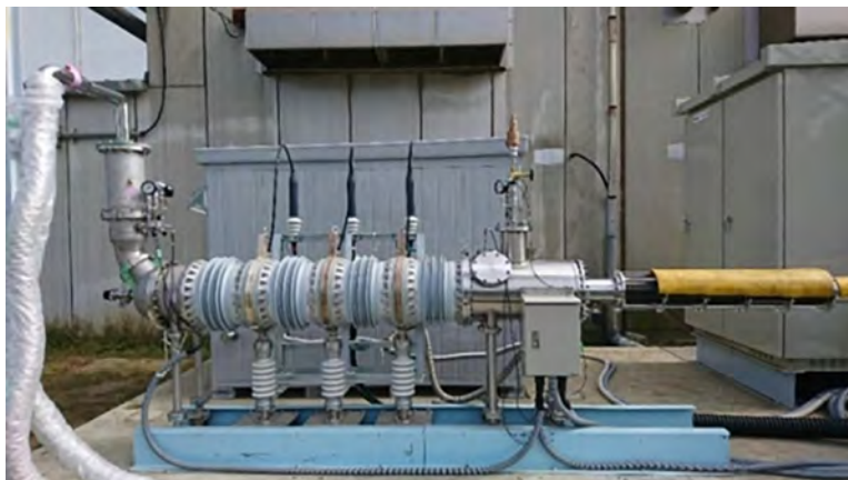
Figure 5. Terminal of tri-axial superconducting cable. Photo courtesy of NEDO.
