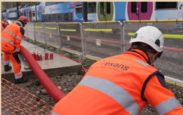
Nexans installs its HTS cable at Montparnasse Station in Paris
