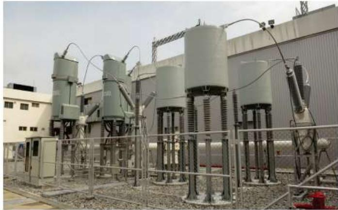
Figure 6. SFCL of 115 kV under commercial service at Glow
