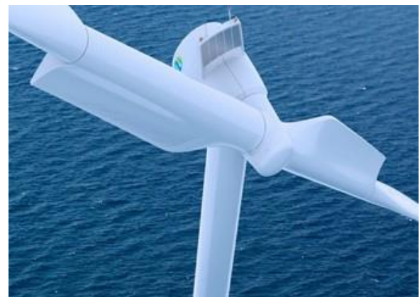
Planning is underway to replace conventional wind generator with HTS based device. Courtesy of EcoSwing.
