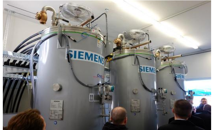
Siemens 10kV Superconducting Fault Current Limiter (Courtesy of Dr. Franz Meyer of BINE Informationsdienst)
