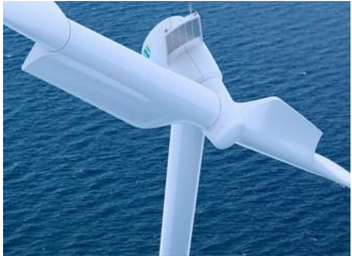
Work is underway to evaluate the possibility to replace large conventional wind generators with HTS-based devices. Image courtesy of EcoSwing.
